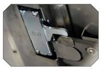
Safe like a vault: 5 mm lock with snap lock and kick guard, 8 mm triangular key.
